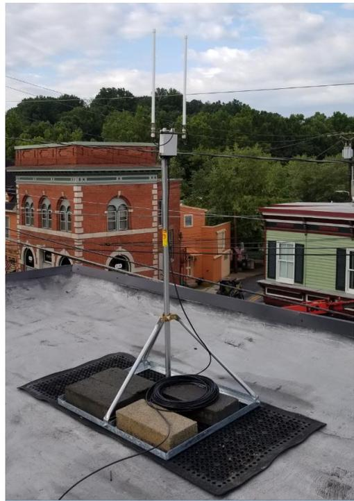
The Fixed Master consists of an outdoor unit (ODU) and an indoor unit (IDU) which are connected together by a Cat5e shielded cable up to 150' long. The IDU has inputs for power (for the ODU), audio (from your streaming audio source), and USB (for the Network Management System). The USB attaches to a PC which runs the Network Management System application.
